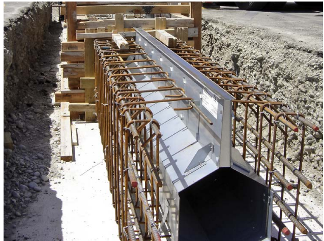
FIG. 1 Christchurch Airport UltraSlot Installation
