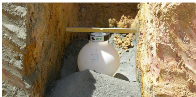
FIG. 1 Smartstream Poo Pit installation on a 160 OD PE line
