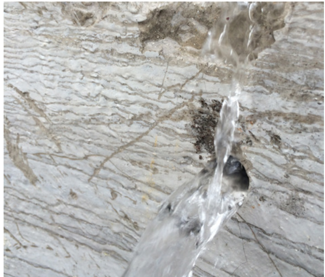
FIG. 1 Leaking MH
