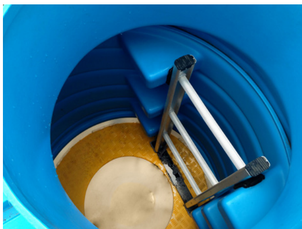
FIG. 1 Smart Pit manhole access view, alloy ladder and bench plate
