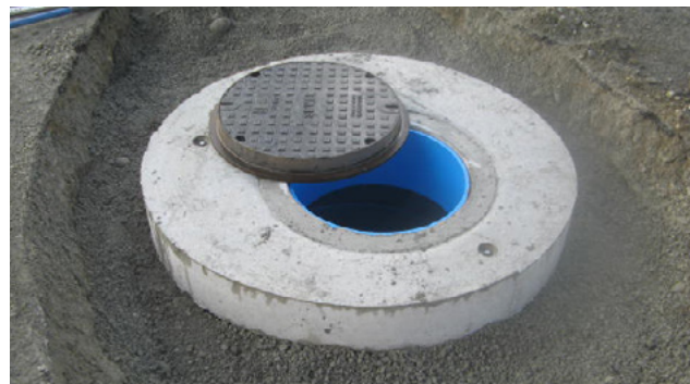
FIG. 2 Precast Concrete Slab and Class D Cover
