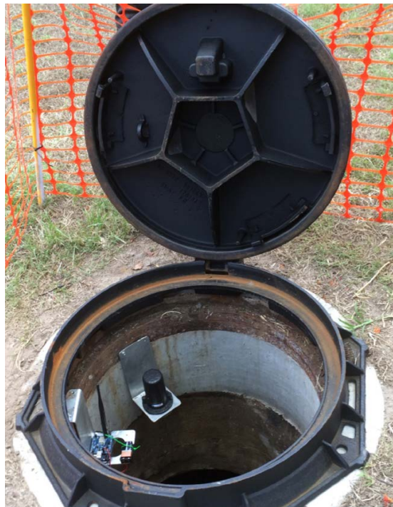
FIG. 2 iCover installation
