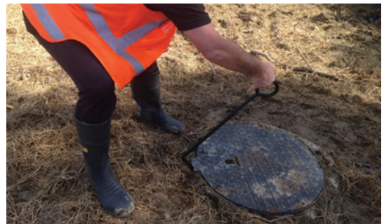
Hook positioned in space between cover and frame opposite hinge
