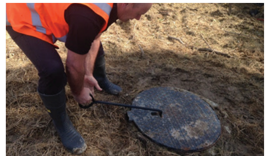
Once 'popped' the bar is then repositioned and the cover lifted
