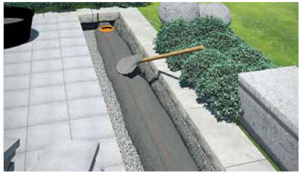
Fill with concrete and compress to foundation.
