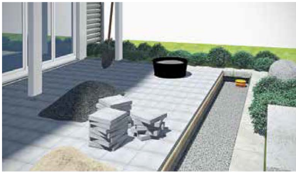
Produce trench in which to lay channel with frost resistant sub base.
